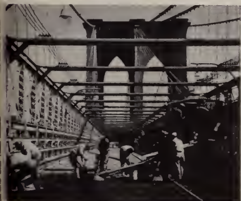
Concrete is poured for the roadway surface on the main span. The view is toward Brooklyn.
